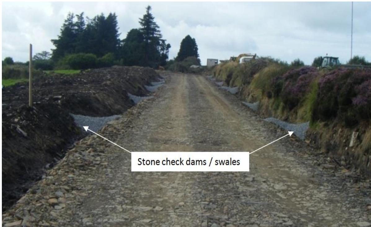
Figure 6-10: Examples of check dams along roadside drainage channels
