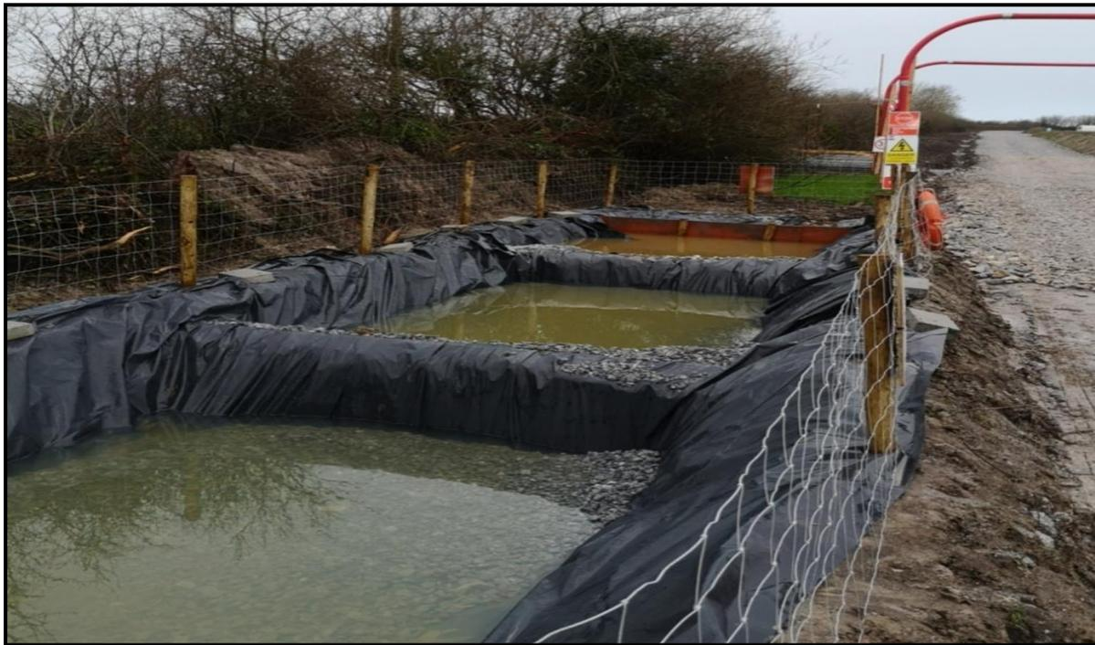
Figure 6-9: Multi-tiered settlement pond with stone filter
